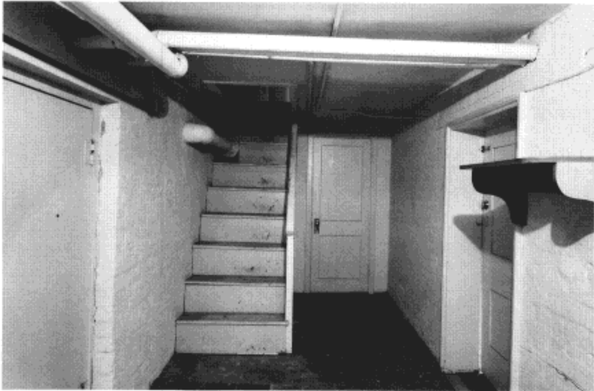
Room B07 Rear stair hall
