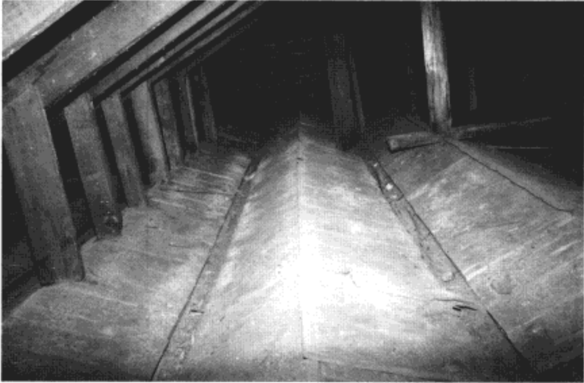
Ridge-and-furrow roof clad with wood boards and tinfoil valleys
