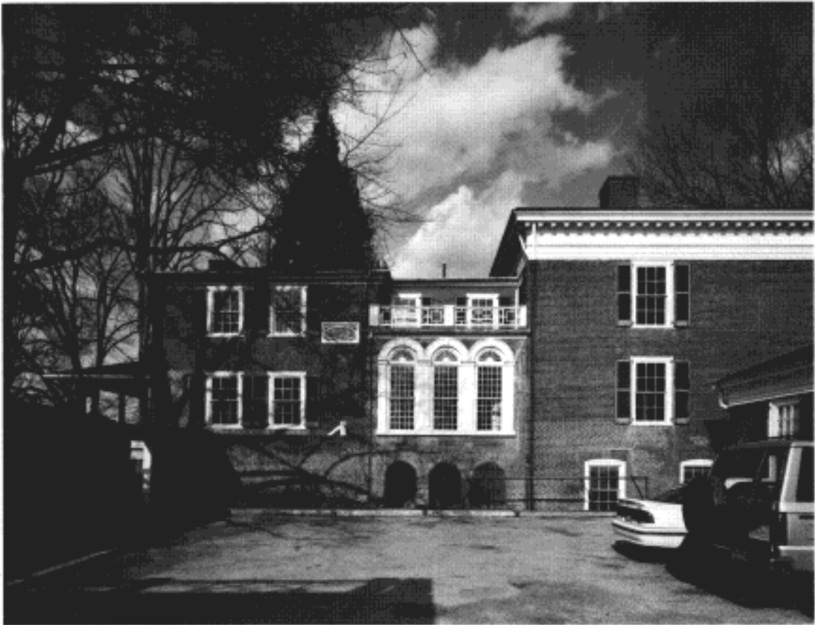
South facade of Pavilion V
