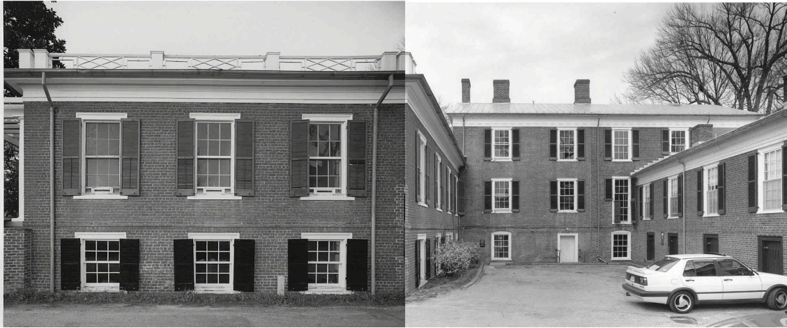
South Façade of Pavilion VII
