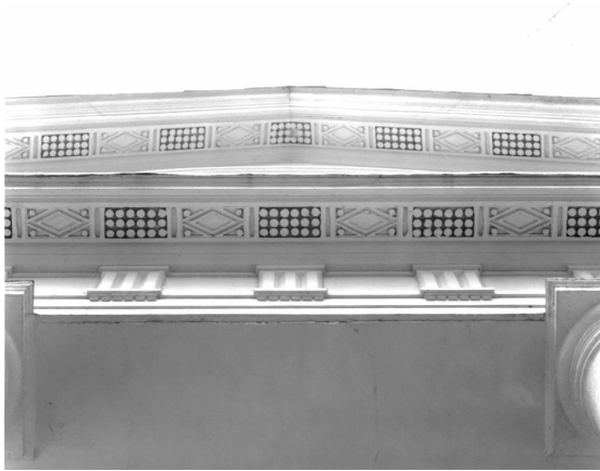
Entablature and column capital at center gable of pavilion
